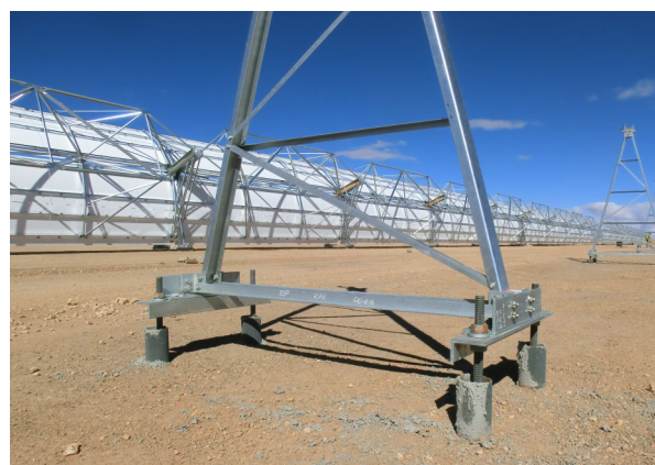
Columns for the parabolic reflector
