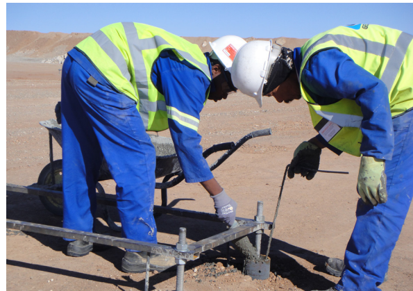
Positioning the bolts
