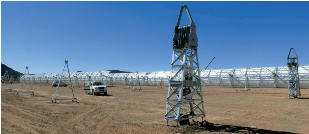
Preparation for the installation of the parabolic reflectors
