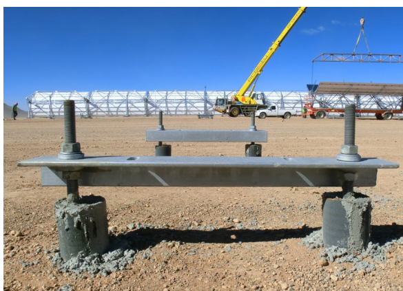
Bolts with substructure
