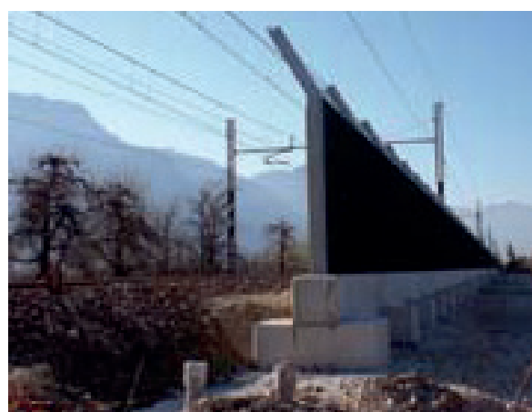
Retaining wall as substructure for the noise protection elements
