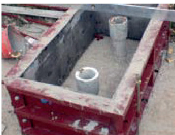
Single foundations with pile distance of 0.75 m.
