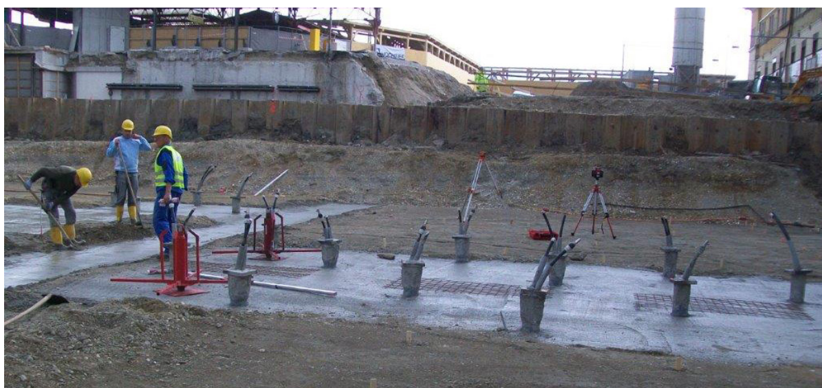
Construction site with installed ductile iron piles and enercret® system
