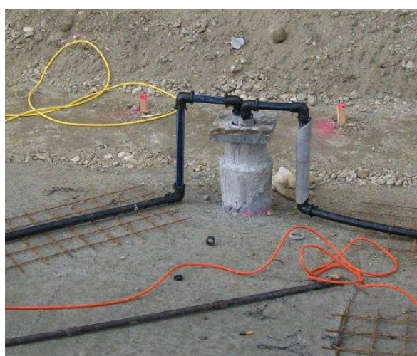
Connection of the absorber pipes
