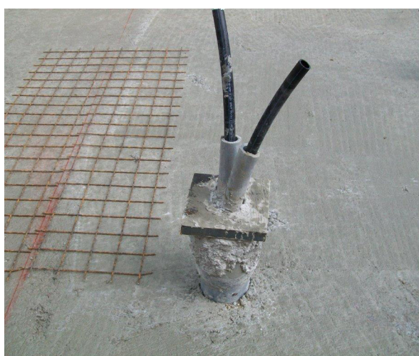
TRM ductile iron pile with the absorber pipes
