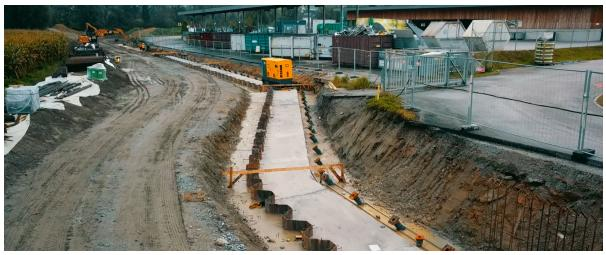
Installed piles are tied into the flood protection concrete foundation
