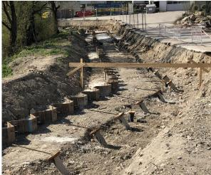
Inclined piles counteract the horizontal forces
