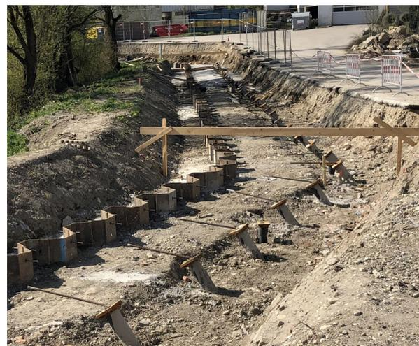
Inclined piles counteract the horizontal forces
