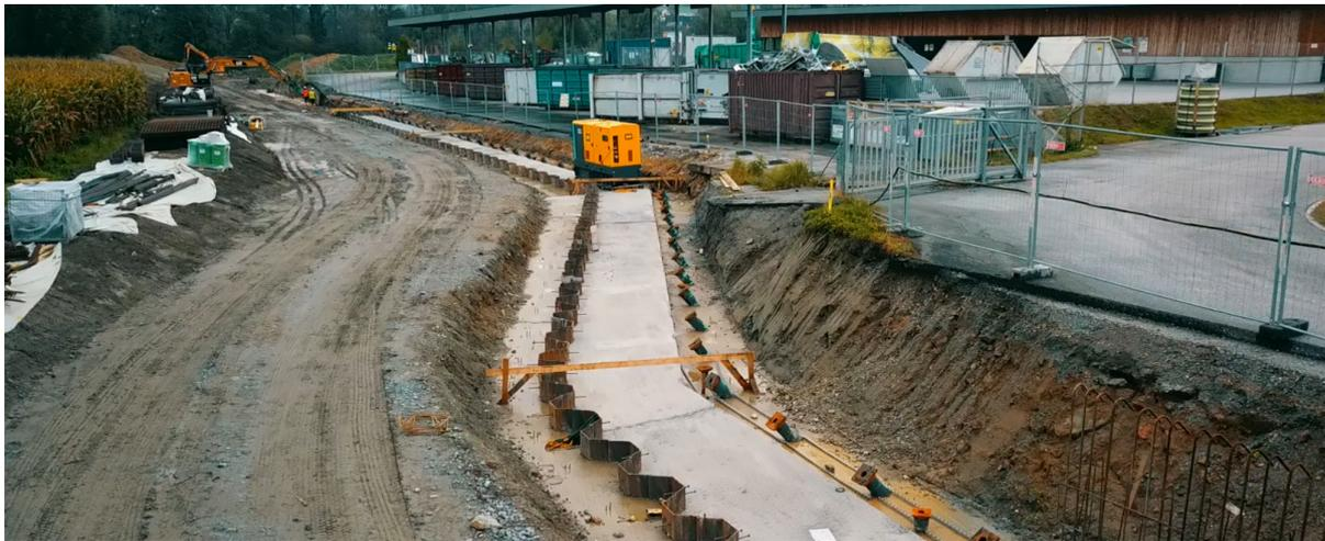
Installed piles are tied into the flood protection concrete foundation
