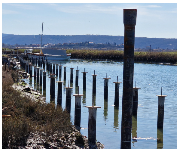
Piles for the jetty
