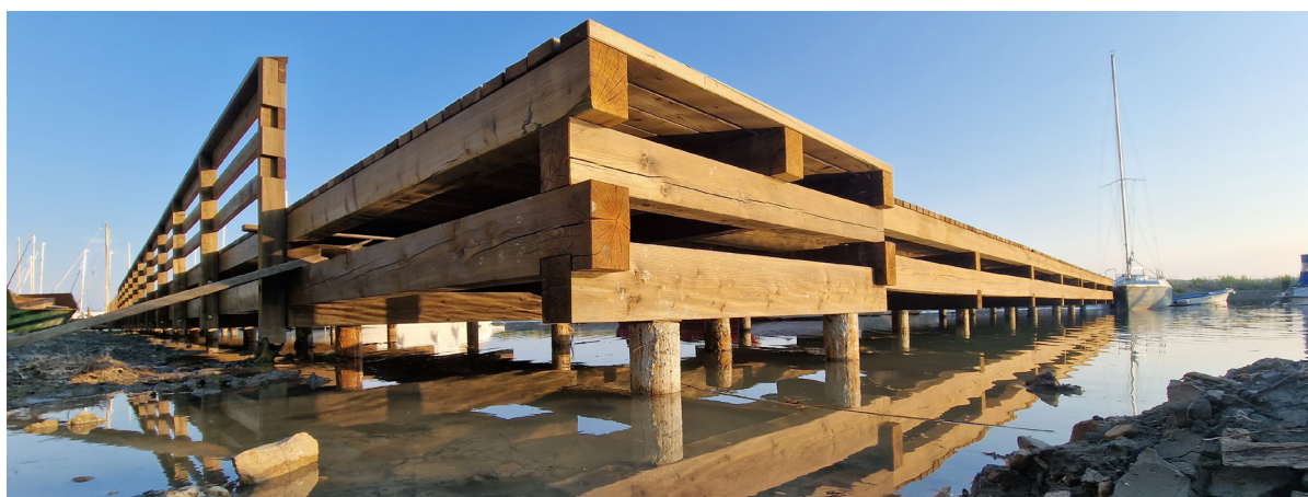
Finished timber pier on ductile iron piles
