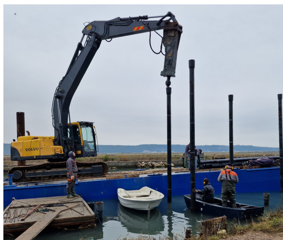
Installation of the piles with excavator
