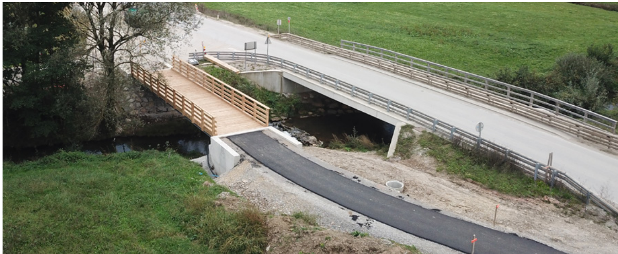
Finished steel/timber bridge standing on non-grouted TRM piles
