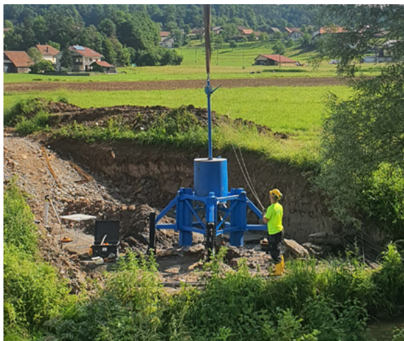
Preparation for dynamic load tests
