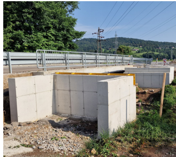
Completed bridge abutments
