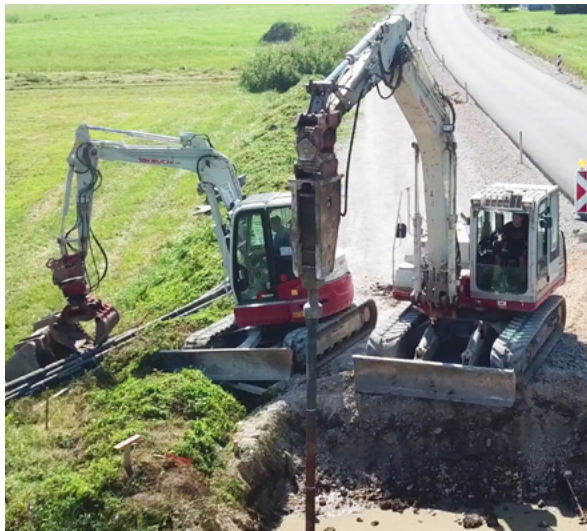
Pile installation
