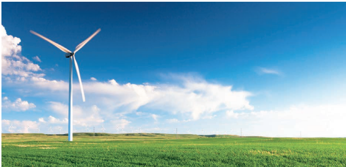
Wind turbines are founded on TRM ductile iron piles.
