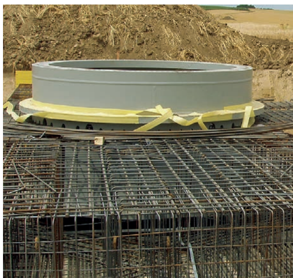
Reinforcement of the foundation
