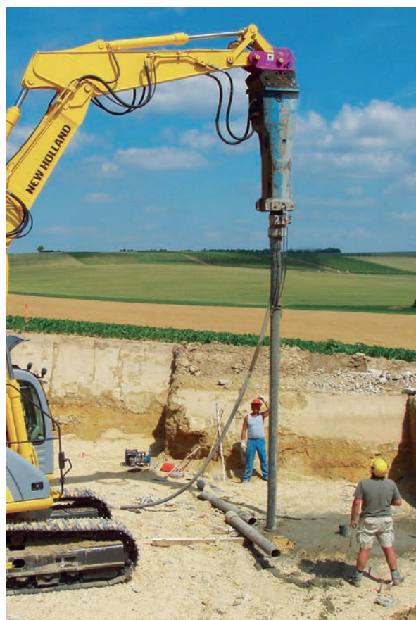
Driving of the grouted ductile iron piles
