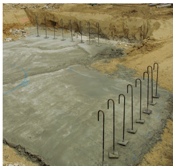
Granular subbase with connection of the tensile reinforcement to the foundation
