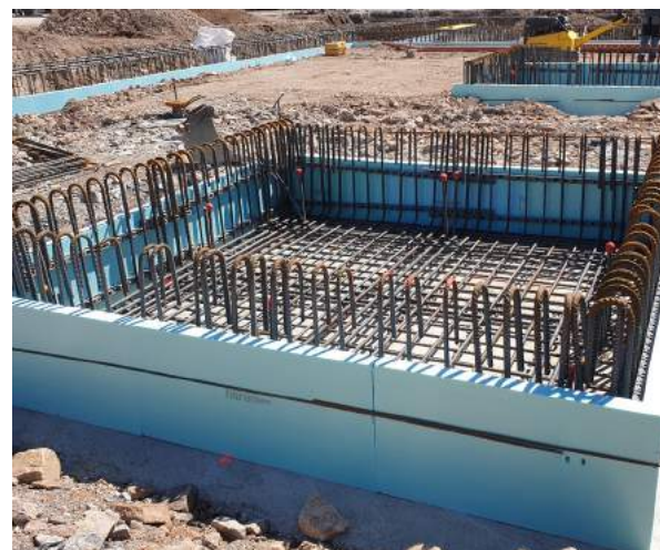
Foundation reinforcement
