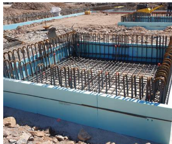
Foundation reinforcement
