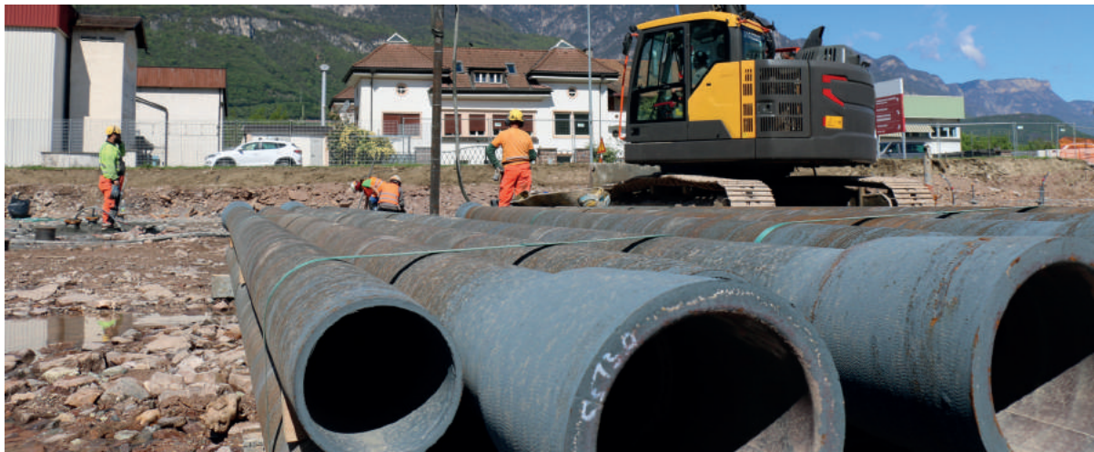
The complete structure stands on TRM piles.
