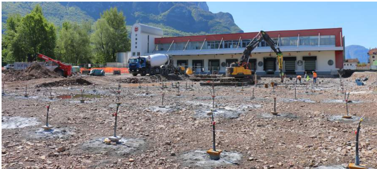
Construction field with installed piles - with geothermal heat exchangers
