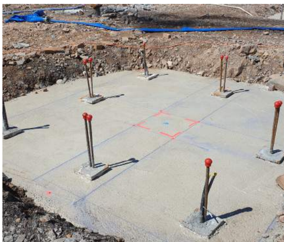
Blinding layer with pile head plate
