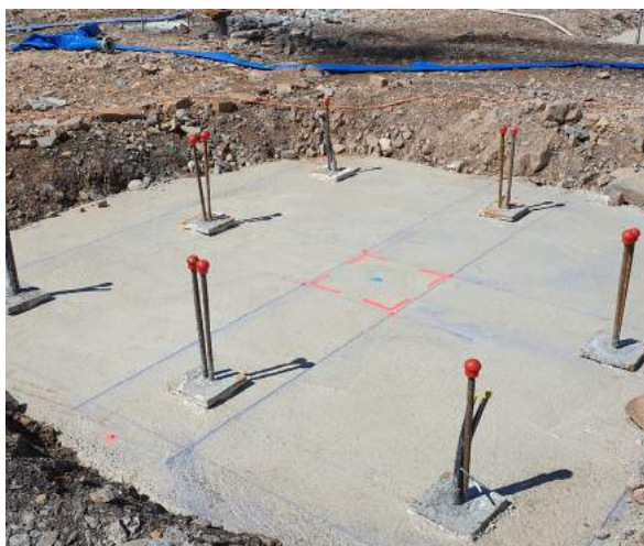
Blinding layer with pile head plate
