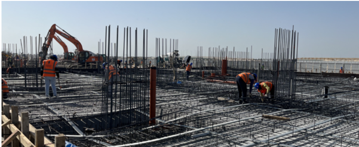
Reinforcement of the CPP
