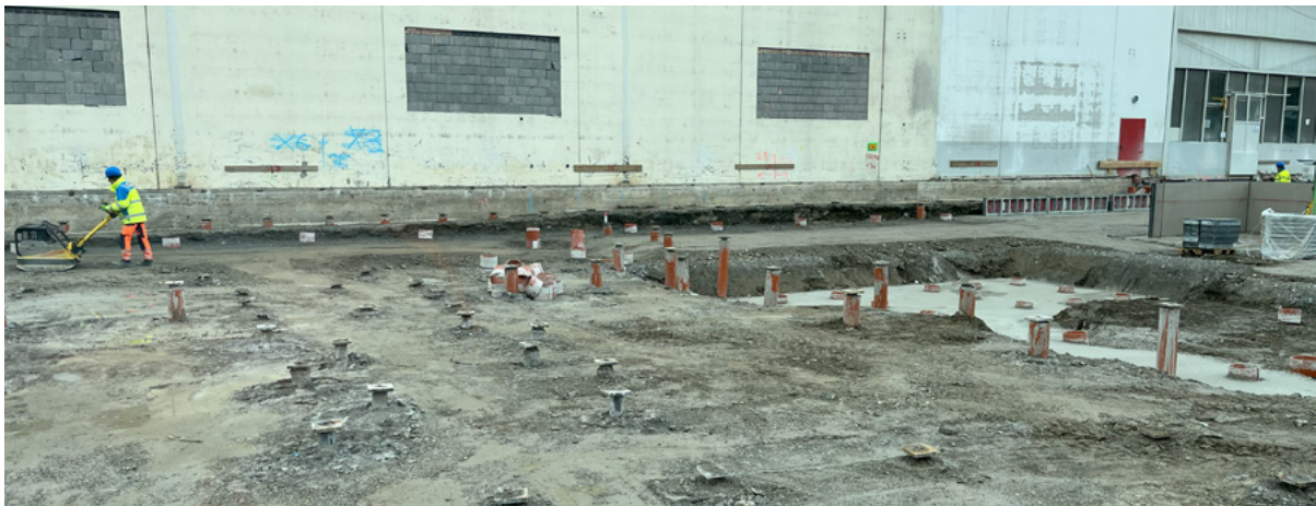
Foundation made of TRM ductile iron piles
