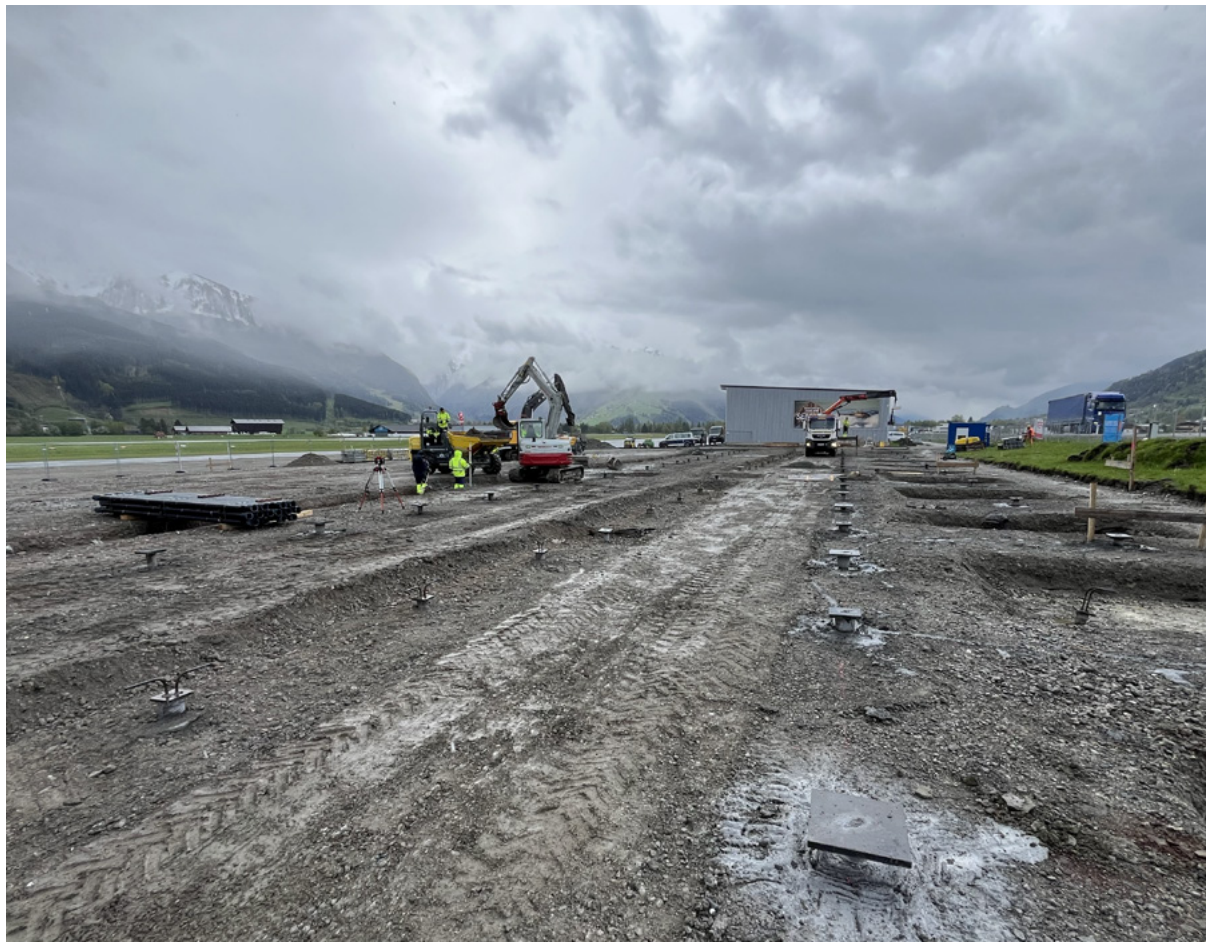
Foundation with TRM Piling Systems
