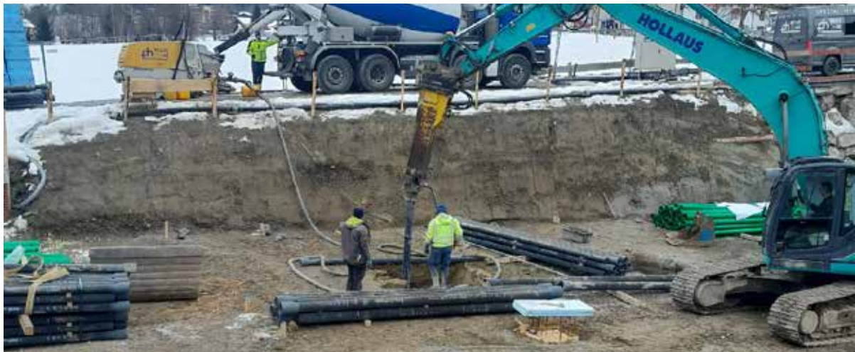
Deep foundation using ductile driven piles
