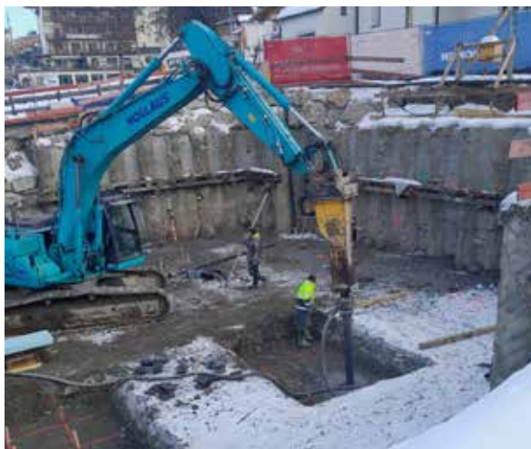
Installation of isolated foundations after pre-excitation
