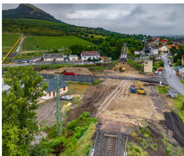
Repair work after the heavy rainfall
