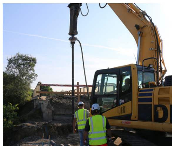
Installation of the TRM ductile driven pile
