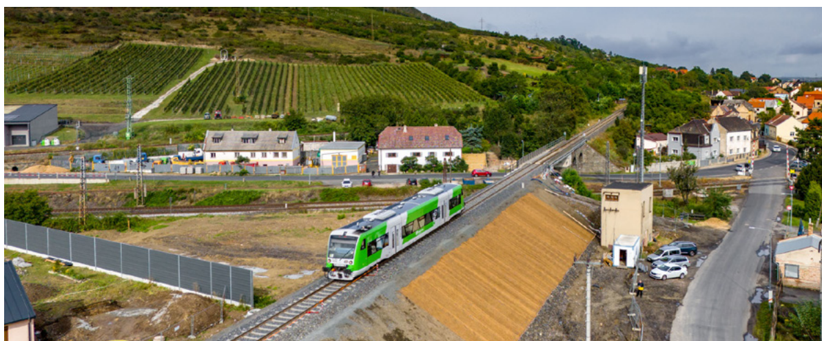
Finalized railroad founded on TRM Piling Systems
