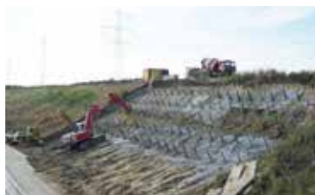
Slope reinforcement
