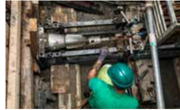
Trenchless laying methods
