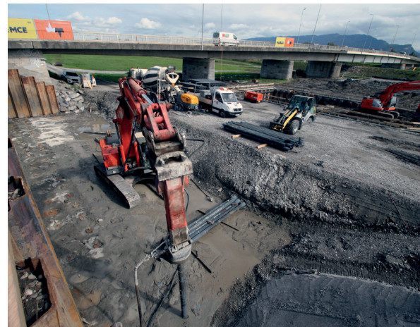
Old Rhine bridge and installation of abutment piles
