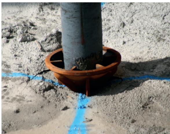
Pile shoe conical grouted
