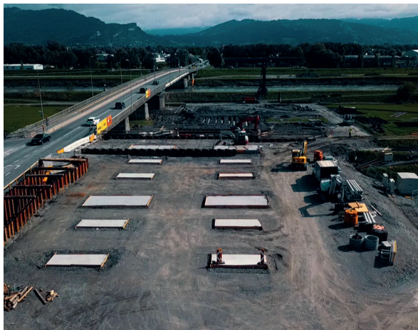
Foundations for bridge insertion
