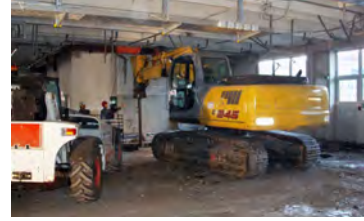
Retrofit foundations with reduced working headroom space
