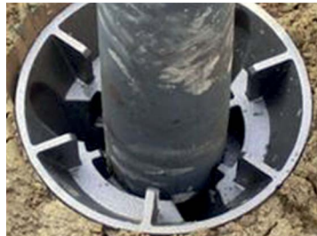
Grouted pile shoe
