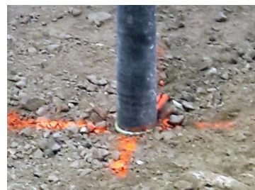
Non-grouted pile shoe
